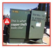
Once the neutral copper is stolen, customers may find that even though their power is on it fluctuates, electronics spark, or arc around the meter box or transformer. Copper thieves often leave open the transformers housed in the green metal boxes containing electrical equipment and live wires. **Touching such transformers could be deadly. Stay away, never touch this equipment, and report it to PNM immediately by calling 888-DIAL PNM.**
